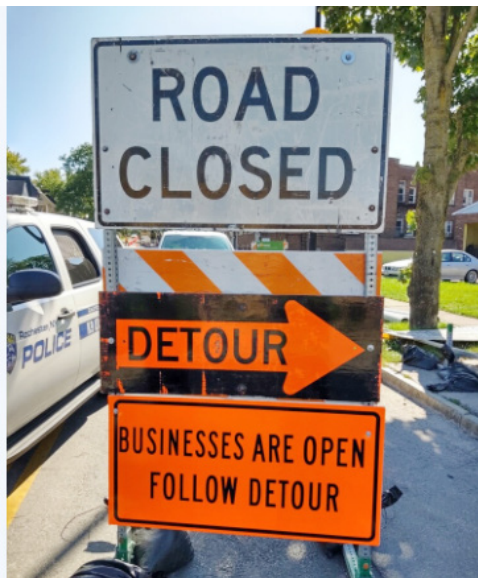
Genesee Street duct bank work.
